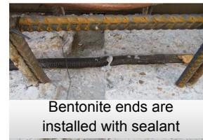
Bentonite ends are installed with sealant
