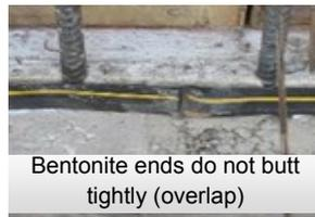
Bentonite ends do not butt tightly (overlap)
