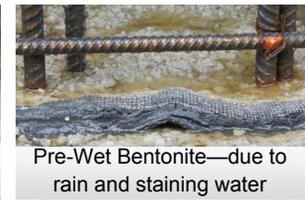
Pre-Wet Bentonite—due to rain and staining water
