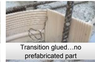
Transition glued...no prefabricated part
