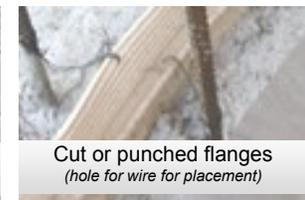
Cut or punched flanges (hole for wire for placement)
