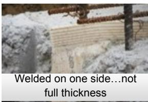
Welded on one side...not full thickness
