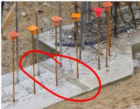
Discuss any footing depressions that will be created due to rebar, base plate, or other component... these will need to be ground down smooth for the installation of a bentonite system.
