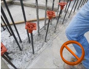
Review the concrete finish requirements with the concrete foreman... bentonite requires a relatively smooth base for proper installation.
