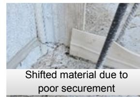
Shifted material due to poor securement
