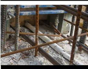
Make sure that the bentonite waterstop is protected during construction... This is a 1/2 pipe covering the bentonite, protecting from water.
