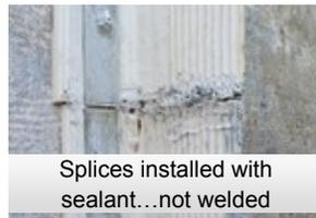
Splices installed with sealant...not welded
