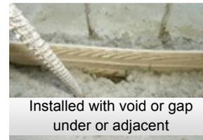
Installed with void or gap under or adjacent
